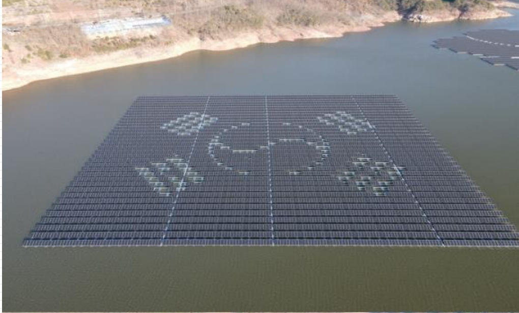
2024 South Korea Imha dam 47MW Floating Solar
