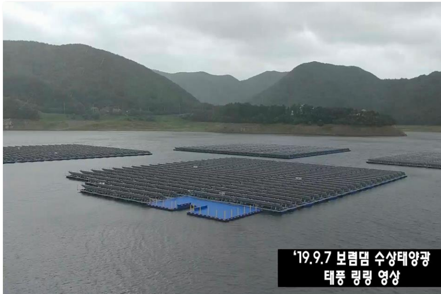
Boyerong Dam 2MW
