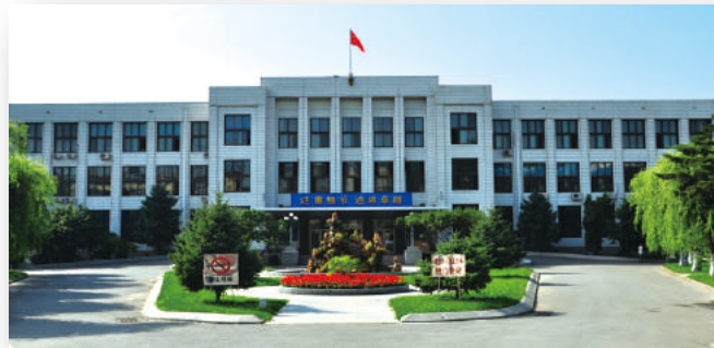
HVRI Old Building
