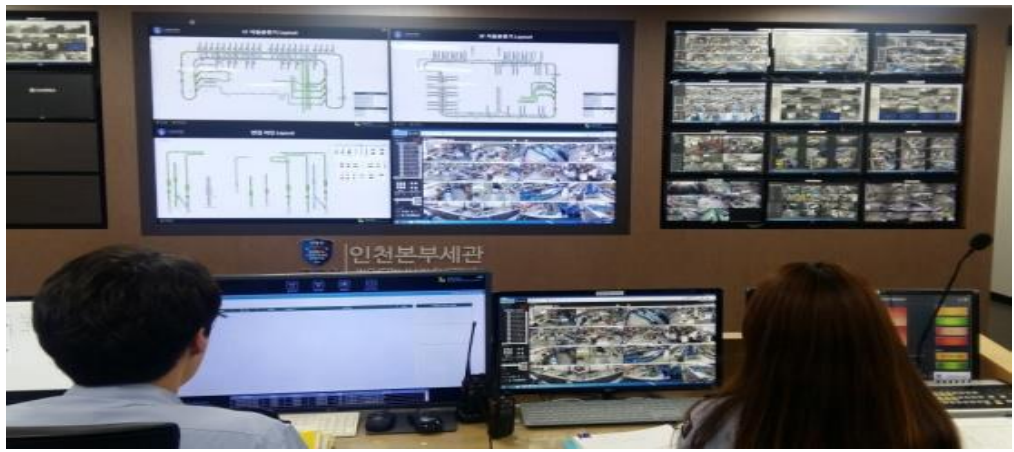
Integrated Control Room
