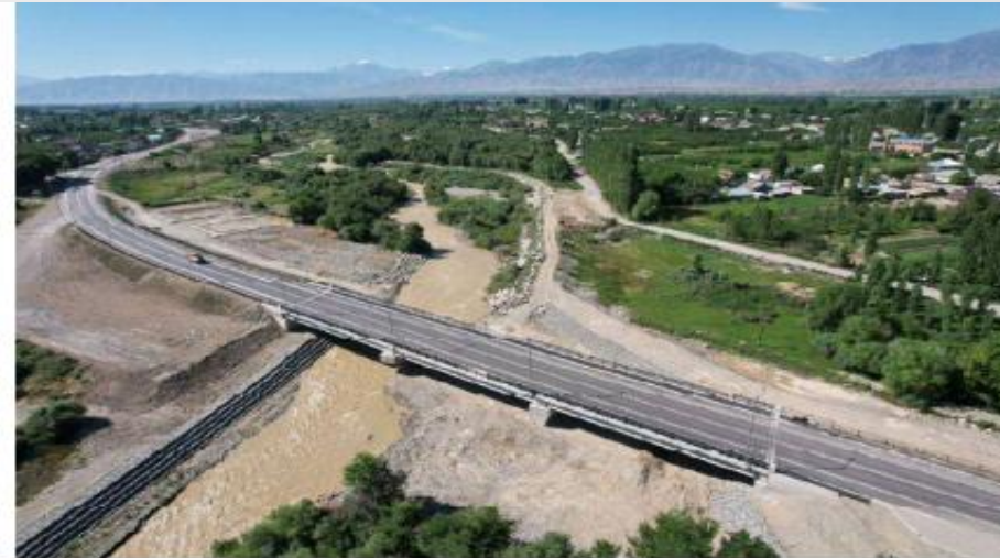
The new bridge
